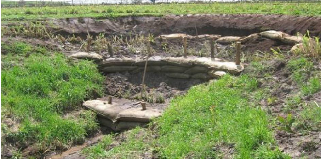
Figure 10: Treatment of gully from head, Source, Nile Basin Initiative, 2012
