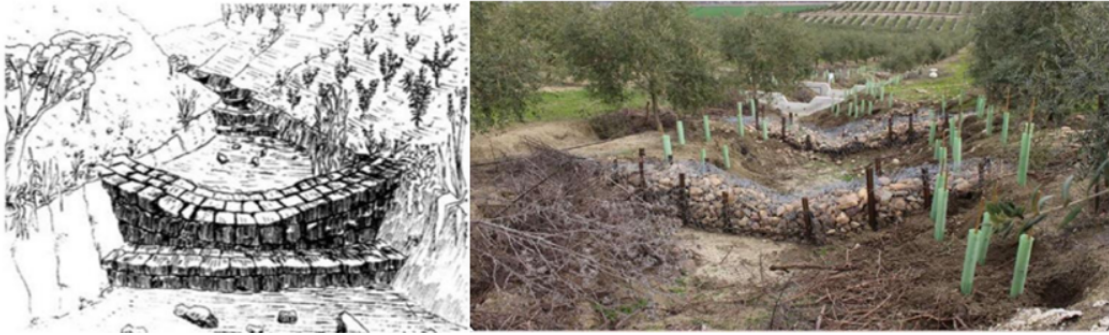
Figure 12: Stone Chekdam, Source Nile Basin Initiative, 2012
